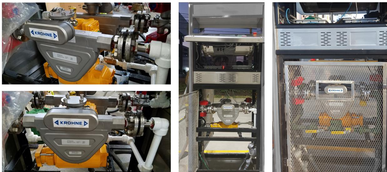
Installation and commissioning of OPTIGAS 4010 Coriolis mass flowmeters for LPG
