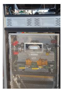
Installation and commissioning of OPTIGAS 4010 Coriolis mass flowmeters for LPG
