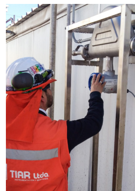
Installation of the flowmeter
