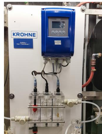
OPTISYS CL 1100 for pH- and temperature-compensated chlorine measurement
