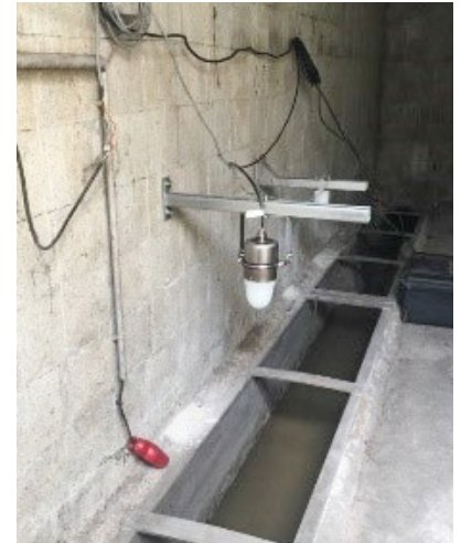
OPTIWAVE 1400 suspended above the open channel
