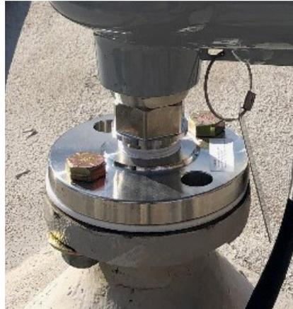
Installation of level transmitter with PTFE sealing between flange and Lens antenna
