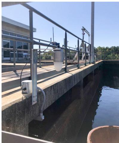
FMCW radar installed next to the overflow pipe
