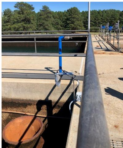
Radar level measurement of water basin
