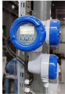
Field-mount converter of the KROHNE Coriolis mass flowmeter
