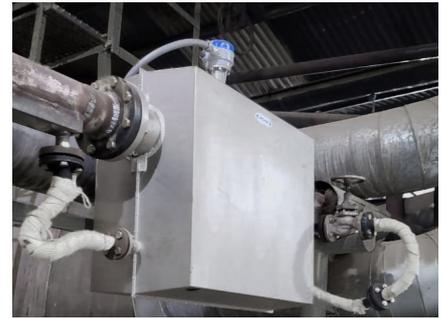
Flow sensor of OPTIMASS 6400 F with integral heating jacket
