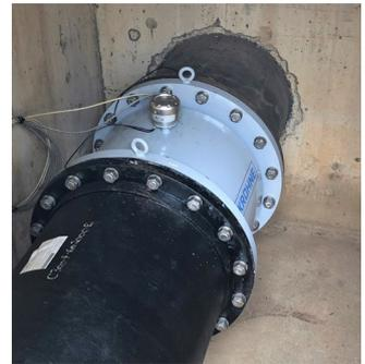
Infeed water measurement with the OPTIFLUX 2300 W
