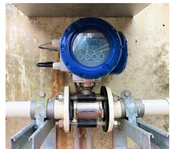
Flow measurement of aluminium sulphate with the OPTIFLUX 7300 C
