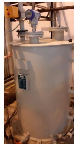
Level measurement of HCl with the OPTIFLEX 7200
