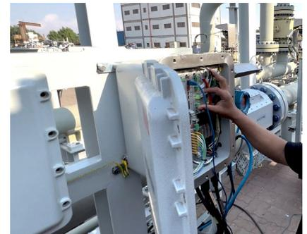
Connecting the remote converter of the ALTOSONIC 5 with a pressure transmitter
