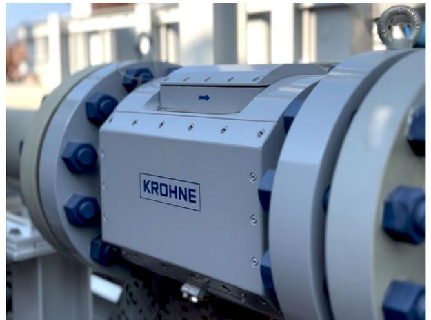
ALTOSONIC 5 flowmeter installed on custody transfer metering system for crude oil
