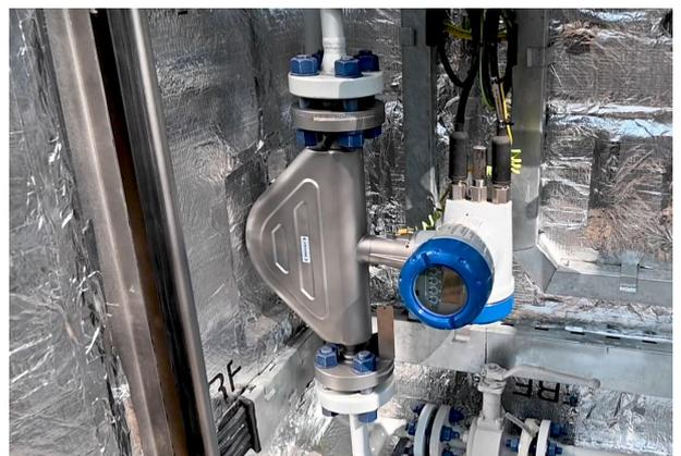
OPTIMASS 6400 Coriolis mass flowmeter mounted on the sampling system
