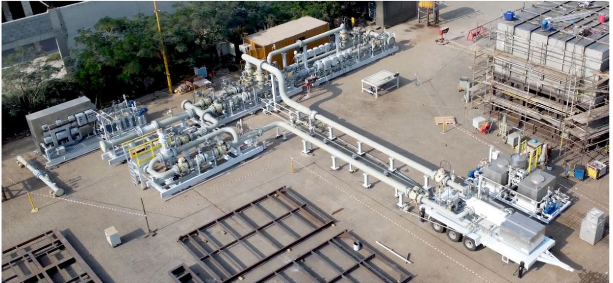
Custody transfer metering system for crude oil with mobile prover and automatic sampling system
