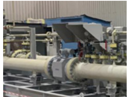
ALTOSONIC V12 for fiscal metering of sour gas
