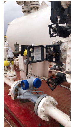
Gas flow measurement on a mobile test separator with OPTISONIC 7300
