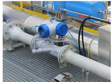
Flow measurement of hydrogen with the OPTISONIC 7300 ultrasonic flowmeter
