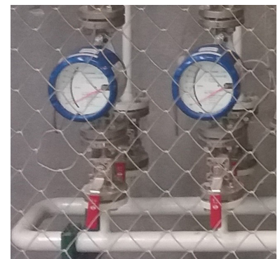
Flow measurement of sulphur dioxide with the H250 M40 flowmeter
