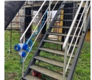
Remote installation of field-mounted signal converter of OPTISONIC 6300
