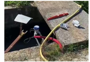
Installation of OPTIWAVE 1540 above irrigation channel
