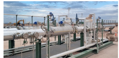
LACT system with KROHNE twin straight tube Coriolis flowmeter
