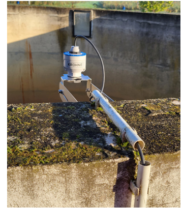
Monitoring the level of a process water storage tank with OPTIWAVE 1540
