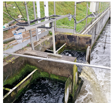
Open channel flow measurement with the OPTIWAVE 1540
