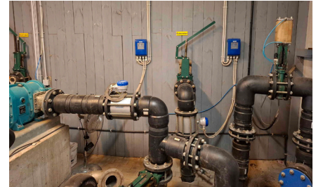
OPTIFLUX 1100 flowmeters measuring liquid manure at a biogas plant
