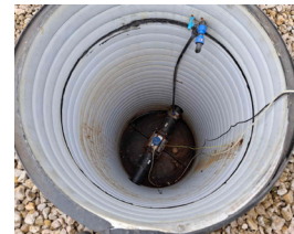
KROHNE electromagnetic flowmeter for manure intake measurement, installed in a well
