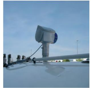
OPTIFLEX on CO<sub>2</sub> tank
