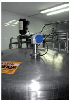
The volume contained in the tank is continuously measured and displayed (in real time) by the OPTIWAVE 7300 C. The OPTIWAVE 7300 C radar level meter was especially designed for liquid products and works according to the non-contact FMCW principle (Frequency Modulated Continuous Wave).
