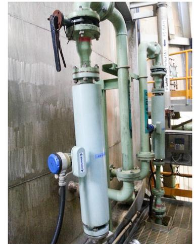
Lime slurry measurement with the OPTIMASS 7400 F
