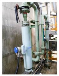
Lime slurry measurement with the OPTIMASS 7400 F
