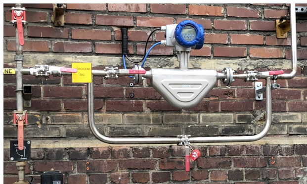
Hydrogen measurement at MERSEN with the OPTIMASS 6400 Coriolis mass flowmeter (DN10)
