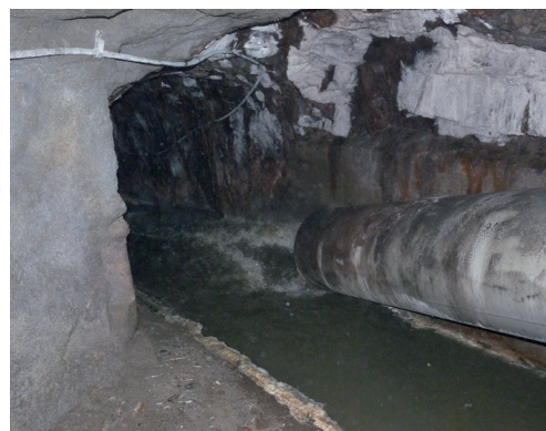
Outlet into wastewater tunnel system
