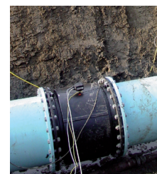
Burial installation of flow sensor
