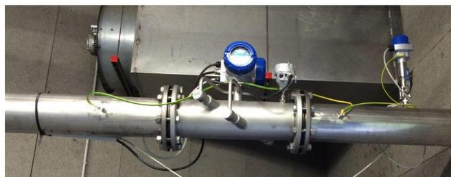
The OPTISONIC 7300 Biogas installed behind the filter
