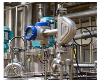
OPTIMASS 6400 dosing edible oil
