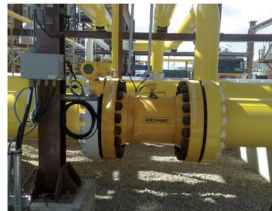
OPTISONIC 7300 unit for flow control in the gas storage process
