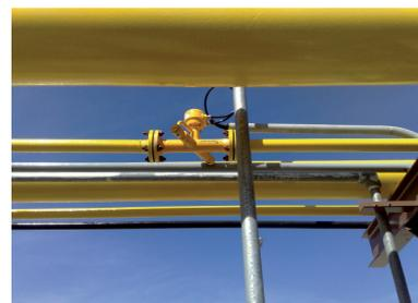
OPTISONIC 7300 unit for measuring the local consumption of natural gas
