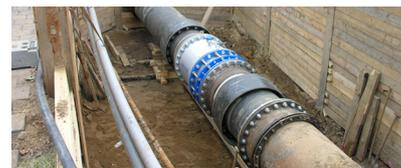
The flange-mounted OPTIFLUX 2300 with virtual reference
