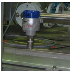
OPTIFLEX 1100 installed on tank
