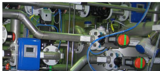
OPTIFLUX 1300 (left and top right), DWM 2000 (right) and OPTIFLEX 1100 (back)
