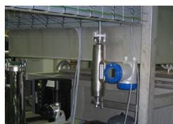
Installation of OPTIMASS 1100 C mass flowmeter
