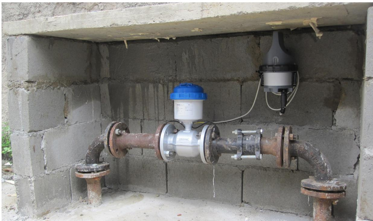
WATERFLUX with GPRS module KGA 42 in aboveground part of the pipeline
