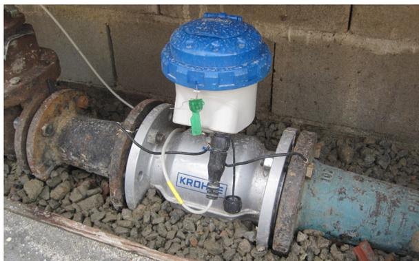
Measuring tube supported by gravel bed
