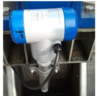
Installation of OPTIWAVE 5200 C with horizontal housing position
