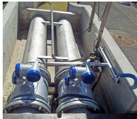
Installation of TIDALFLUX 2300 in sewage channel
