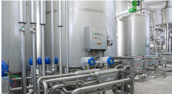
Installation of the OPTIMASS 6400 in front of the buffer tank
