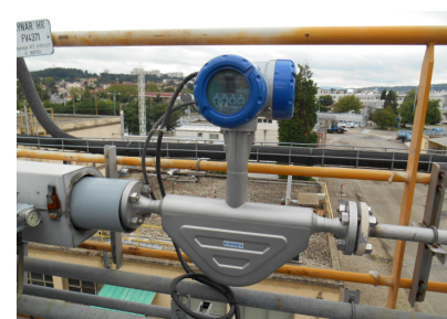
Measuring gas mixture with the OPTIMASS 6400 C
