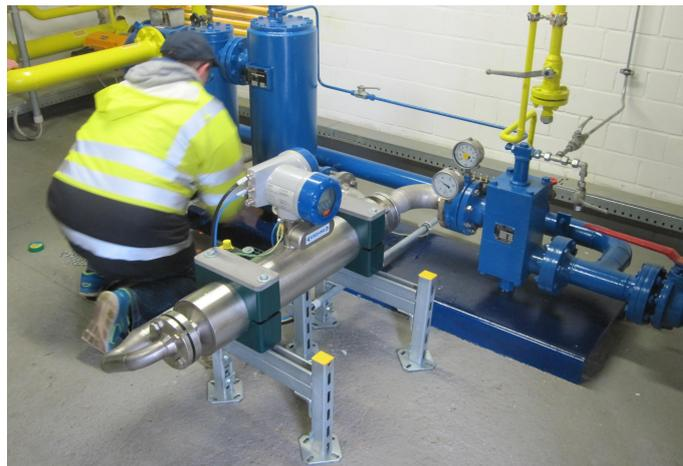
Space-saving installation of the OPTIMASS 7300 C in the measuring facility
