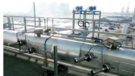
Steam measurement with the OPTISONIC 8300
