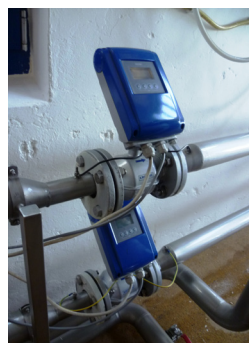
Water flow measurement with the WATERFLUX 3100 C
