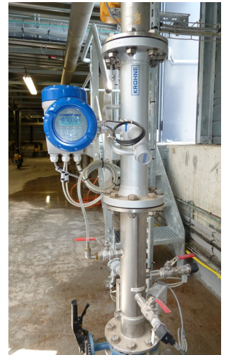
Biogas measurement with the OPTISONIC 7300 C ultrasonic flowmeter
