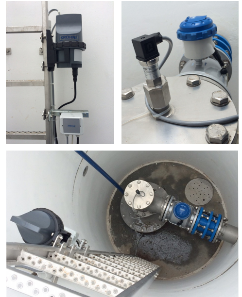
Top left: Data transmission with KGA 42; Top right: OPTIBAR P 1010 C and WATERFLUX 3070 C;
