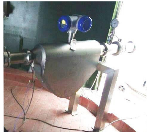
Installation of OPTIMASS 6400 (DN100 / 4") with SMS connections for hygienic flow measurement of bright beer
