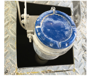
OPTIWAVE 6400 installed on top of the storage silo
