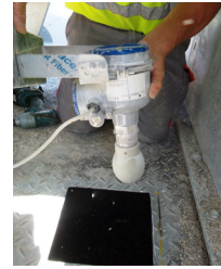
OPTIWAVE 6400 installed on top of the storage silo
