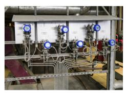
OPTIBAR DP 7060 C Differential pressure transmitter for the zone regulation of the bottom air
