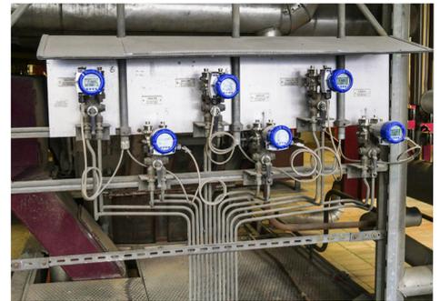
OPTIBAR DP 7060 C Differential pressure transmitter for the zone regulation of the bottom air
