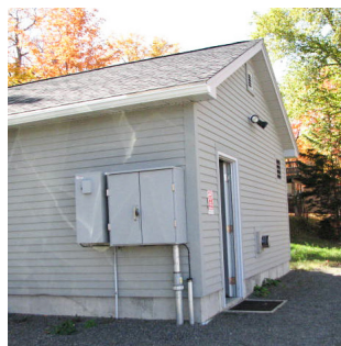
Pump station where the measuring system is installed
