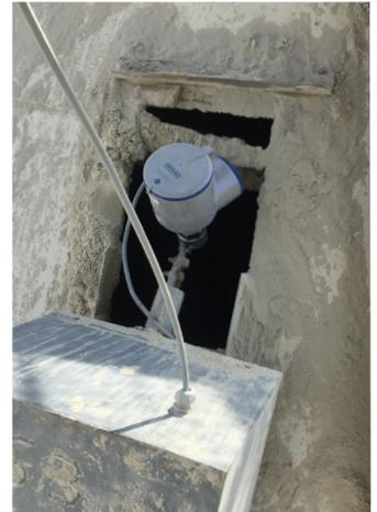
Retrofit with flush-mounted OPTIWAVE 6500 radar level transmitter
