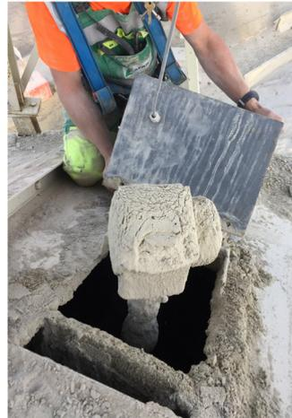
Removal of old OPTIWAVE 6300 level transmitter
