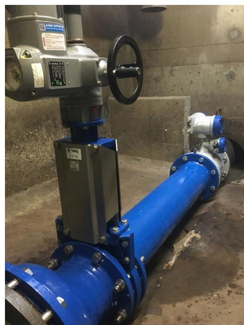
Measuring solution including flowmeter and slide valve
