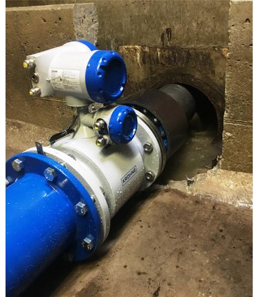
TIDALFLUX 2300 – Flowmeter for gravity pipelines
