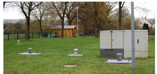
Transfer of measuring signal to the control cabinets
